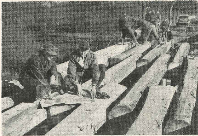
Lt. "Mike" shows his SS foreman the proper position that the next timber goes in the infantry-built bridge over the Kremns River.
